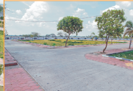
CC Road having pavers both sides
